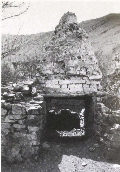
Fig. 3: The collapsing mchod-rten at Alchi Shang-rong (CL94 14,35)
